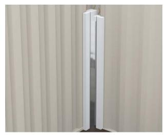
Press the metal insert into the grooves. If the metal is loose, use sprayfoam or duct tape to hold in place.
