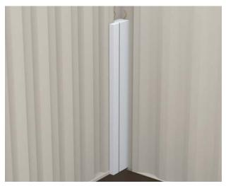
Install the larger insert first in the end wall. Cut out for the diagonal braces in the corner.
