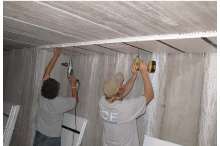
Panels installed with Tapcon screws.
