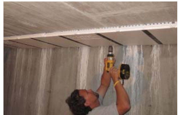
Panels installed with Tapcon screws.
