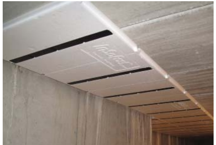
Install ceiling panels first.
