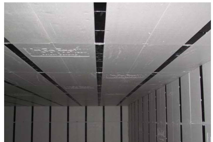
Ready for drywall.
