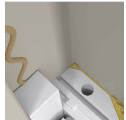
Fill the corner with foam.
