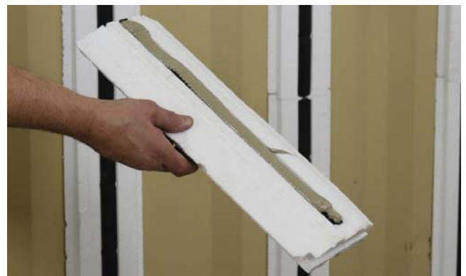
Adhesive on LowPro Insert.
