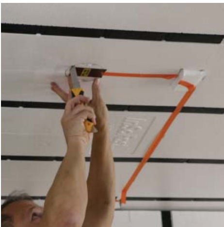
Cutting out for round outlet box.
