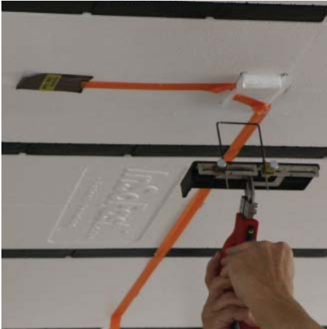
Cutting out raceway intersection.
