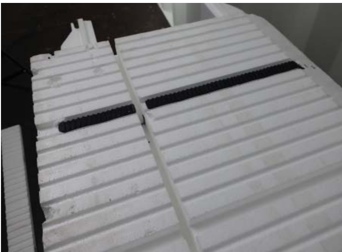
Foam is removed to accommodate the rail.
