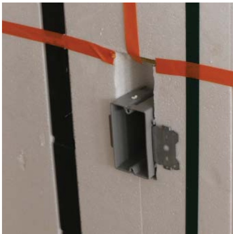
Face mount electrical box makes installation easier.
