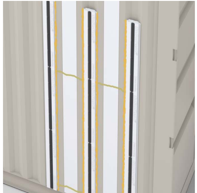
Place PL Premium horizontally and spray foam along the edges.
