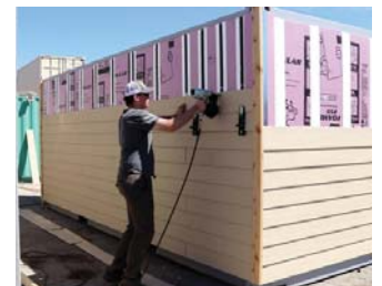
Exterior Siding Pages 22-23
