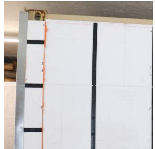
Metal flashing installed for added attachment.
