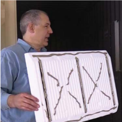
Use plenty of adhesive on the doors.
