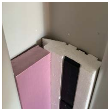
Fill the void in the corners with sheet foam.
