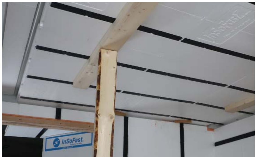
"T" bracing is installed every 4' - Don't pound into place.
