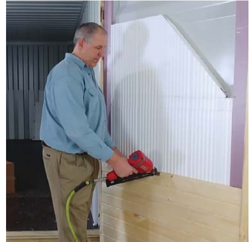
Nailing on cedar siding.
