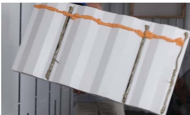
For the first row, use spray foam along the floor or on the bottom of the panel.
