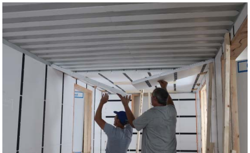
Installing the ceiling panels.
