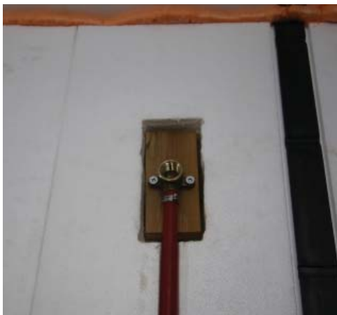
Use recessed 1x3 to secure shower plumbing.
