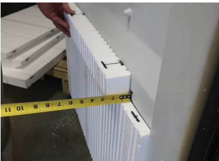
Measure for the thickness needed.
