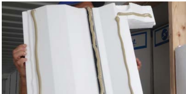
Always add additional adhesive to the back of the panel around openings
