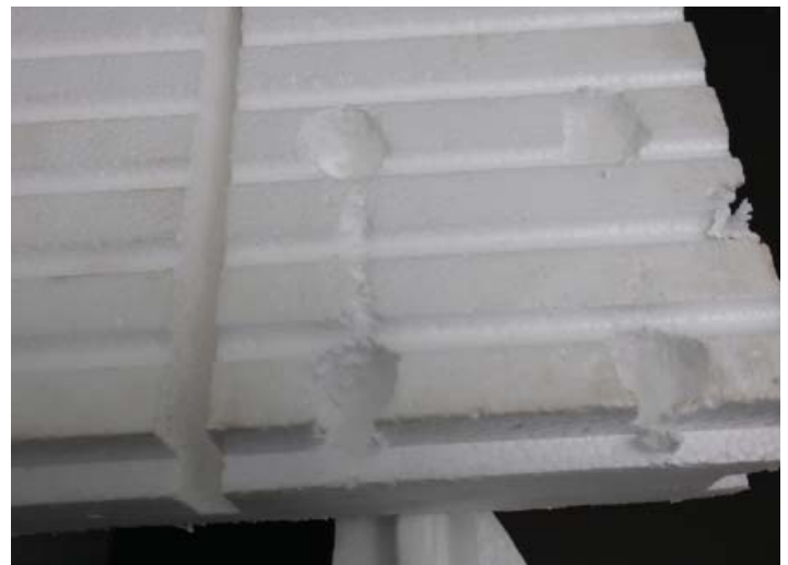
Drill out the foam where the fastener heads are located.
