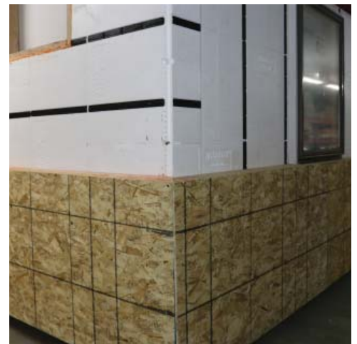
Exterior build out is ready for WRB.
