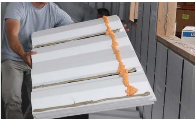
Adhesive and spray foam on CX panels.
