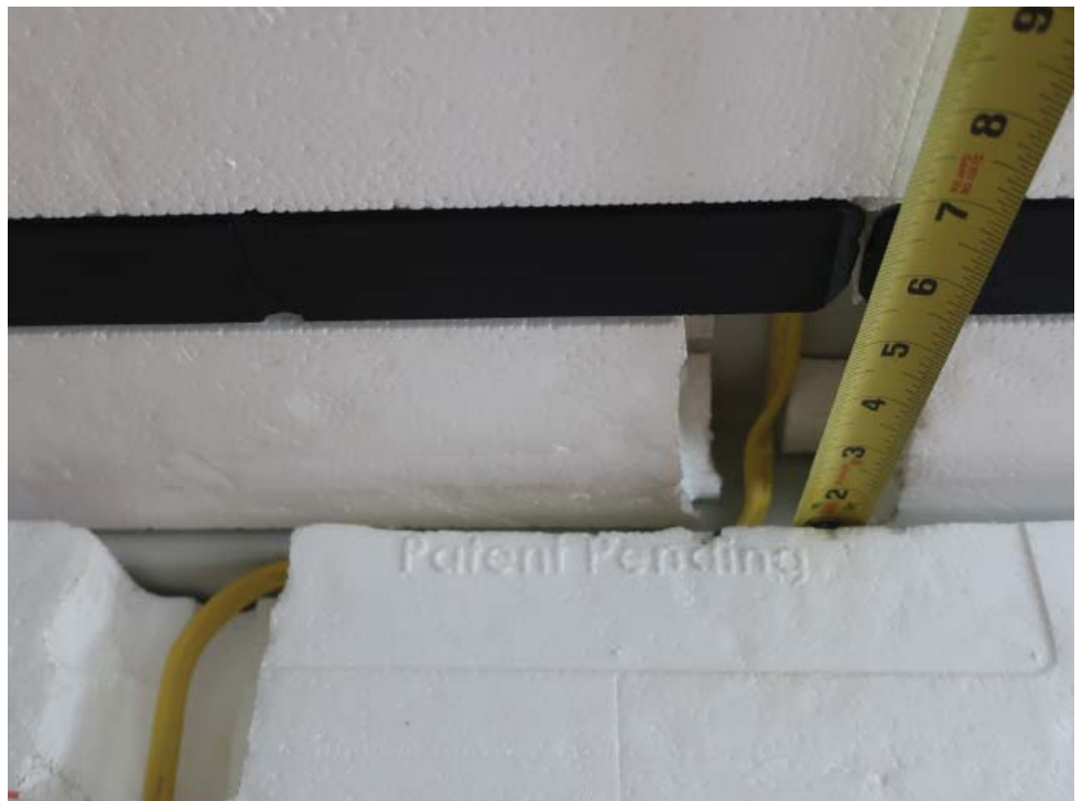
No protective nail plate required provided the wire is a minimum of 1-1/4" back from the surface of the foam.
