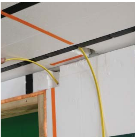
Running wiring down the wall.
