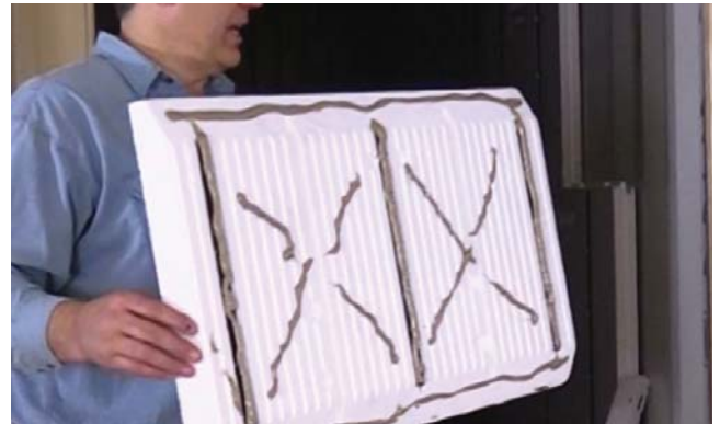
Adhesive on the studs and foam of a flat panel.
