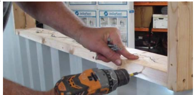
Wood jamb installed.
