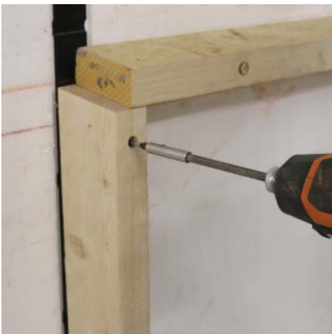
Screw framing into InSoFast stud.
