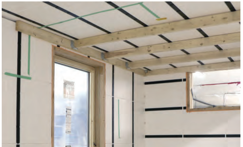
2x4 framework for allows for additional insulation.
