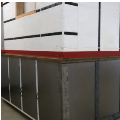
Raw steel was added on lower part of wall.
