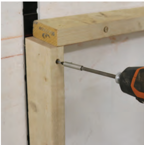
Screw framing into InSoFast stud.
