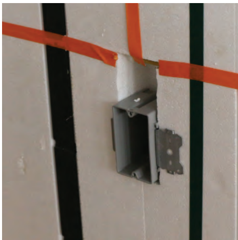
Face mount electrical box makes installation easier.
