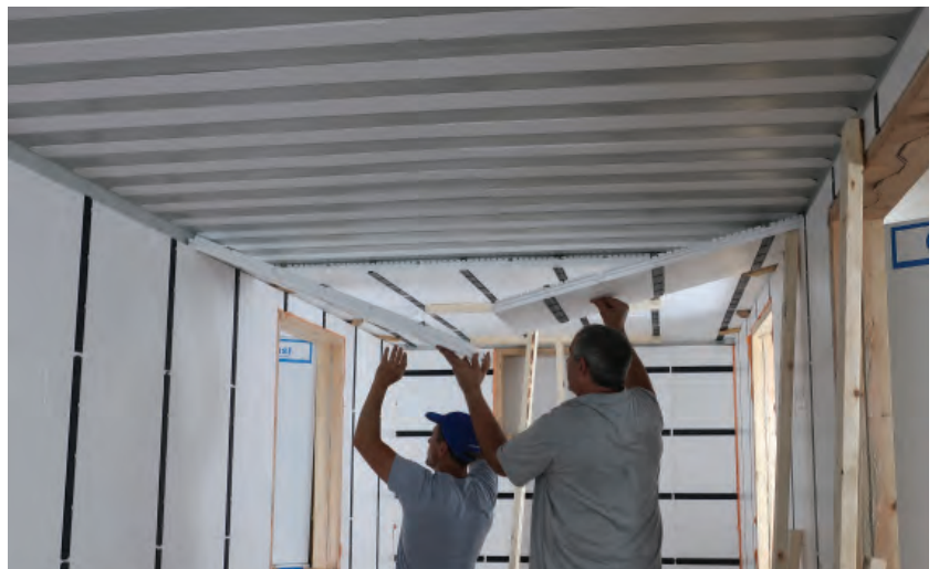
Installing the ceiling panels.
