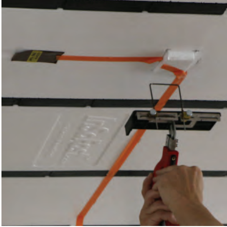
Cutting out raceway intersection.
