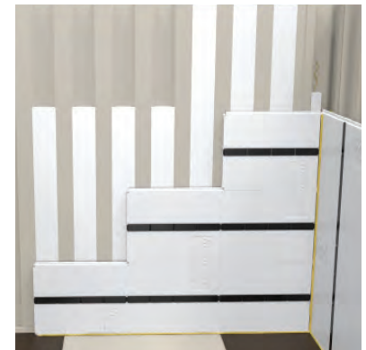
Running bond pattern vertically.
