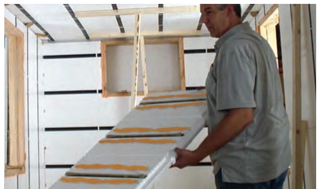
PL Premium plus additional spray foam for ceiling panels.
