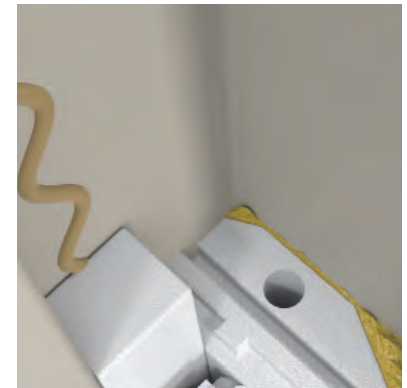
Fill the corner with foam.
