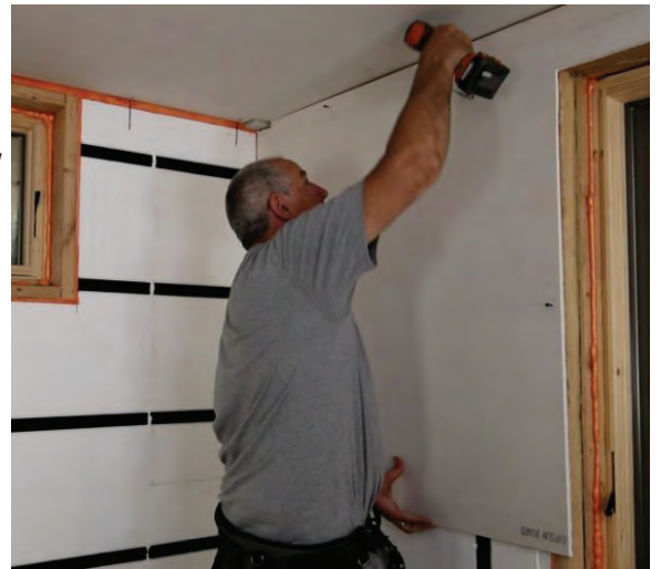
Install drywall using standard drywall screws for wood.
