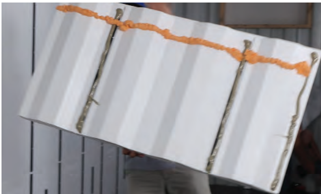
For the first row, use spray foam along the floor or on the bottom of the panel.
