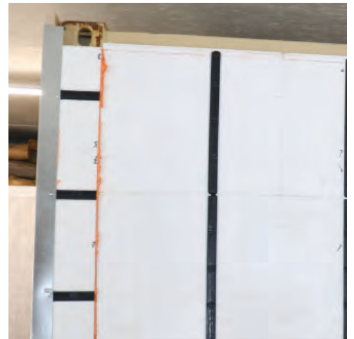
Metal flashing installed for added attachment.
