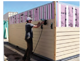
Exterior Siding Pages 22-23
