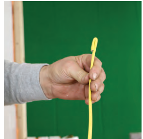
Bend over the tip of with wire when pushing through.
