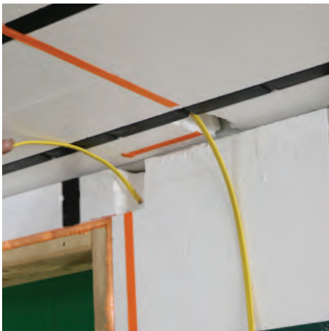
Running wiring down the wall.
