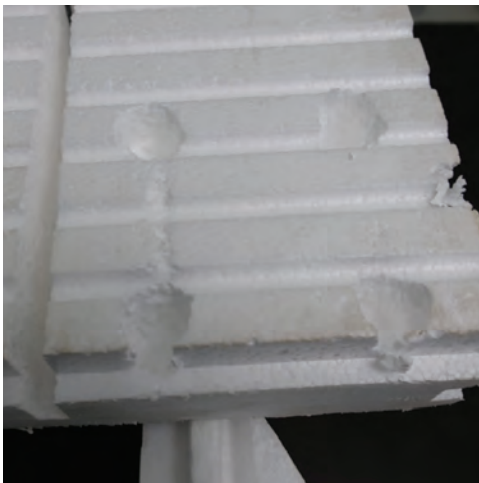
Drill out the foam where the fastener heads are located.
