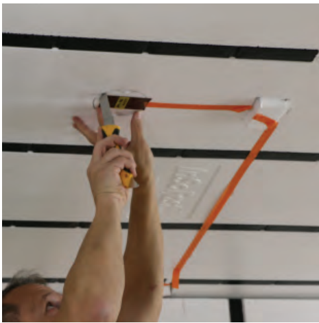
Cutting out for round outlet box.
