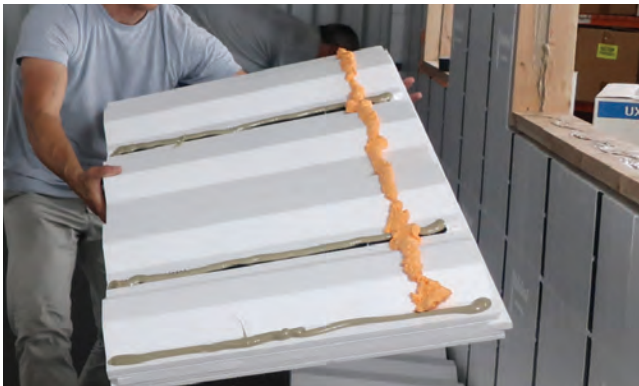
Adhesive and spray foam on CX panels.
