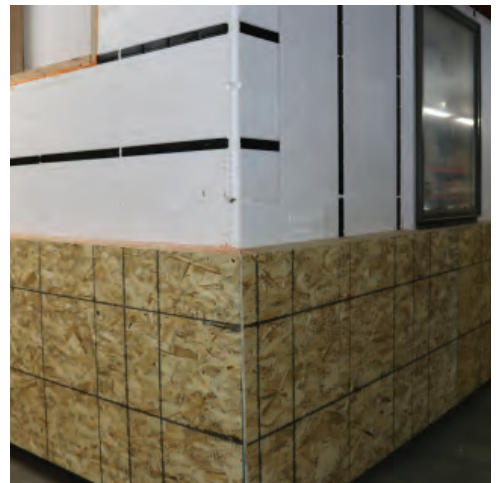
Exterior build out is ready for WRB.
