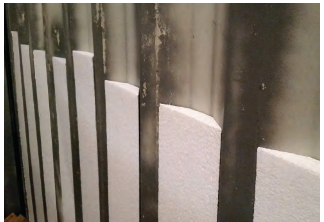
Installing side wall inserts.
