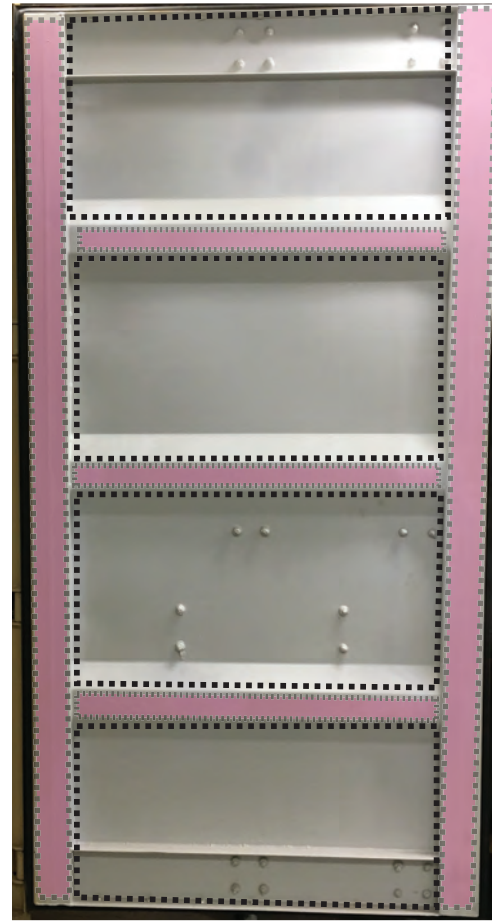
InSoFast panels are used for the middle area and then sheet foam for the pink areas.
