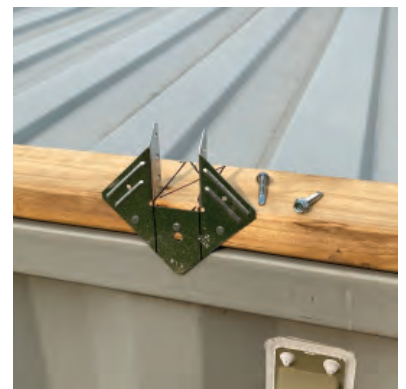
Hurricane anchor to attach roof to container.
