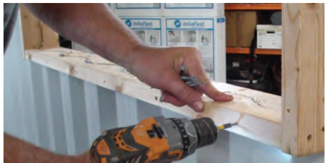
Wood jamb installed.
