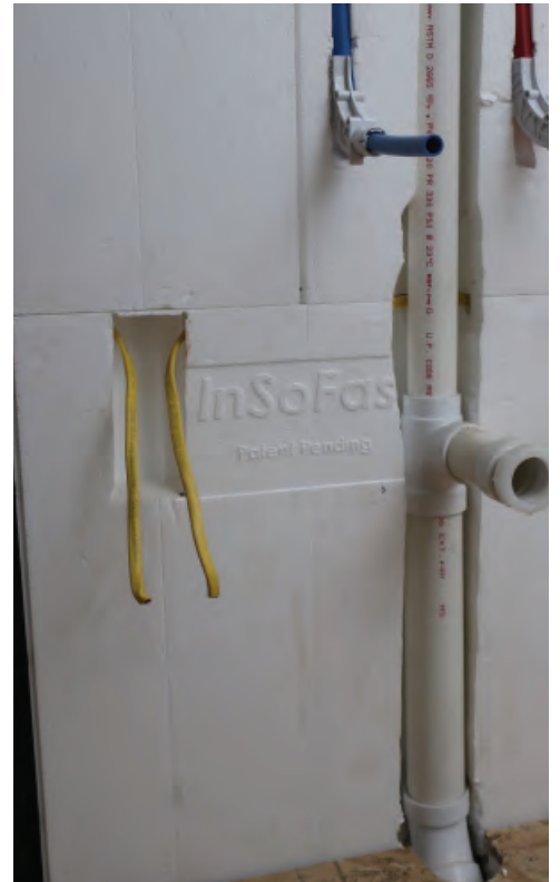
The CX 44 panel can accommodate a 2" PVC pipe.
