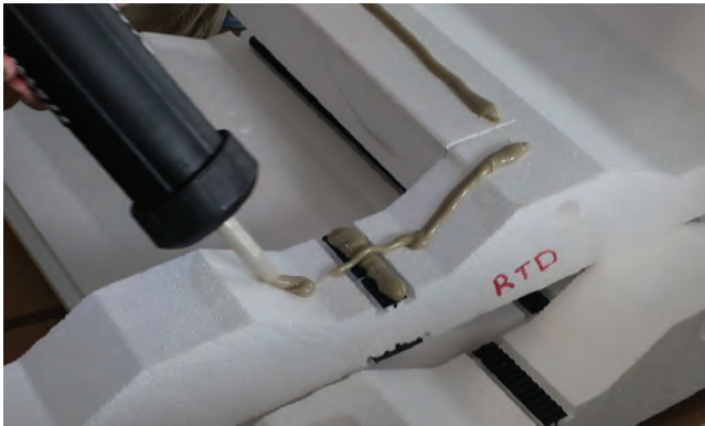
Applying adhesive on stud and around a cut.
