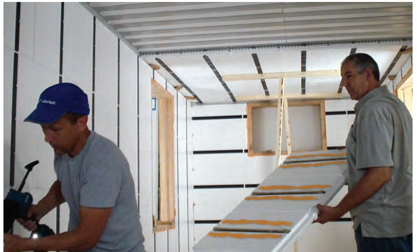
To keep the studs centered in the container, trim off the ends of both panels.
