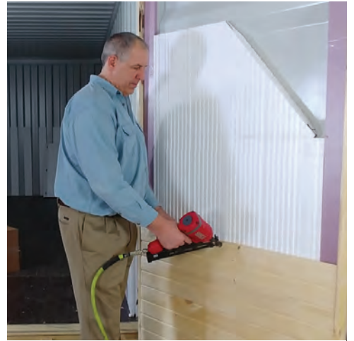
Nailing on cedar siding.
