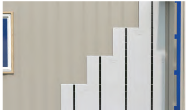
Install the panels in a running bond pattern.
