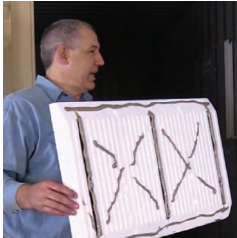
Use plenty of adhesive on the doors.
