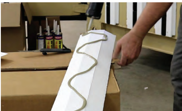
Applying adhesive to side wall insert.
