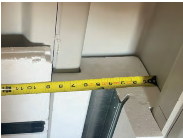
Measure out 8-1/2" along the end wall.
