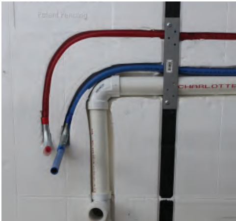
Use protection plates where necessary.
