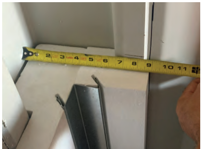
Measure out 9" along the side wall.
