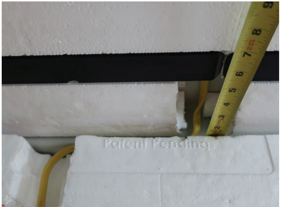
No protective nail plate required provided the wire is a minimum of 1-1/4" back from the surface of the foam.
