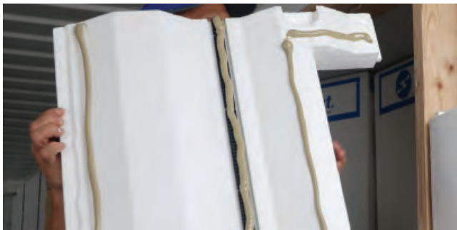
Always add additional adhesive to the back of the panel around openings
