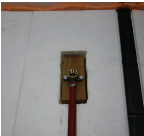
Use recessed 1x3 to secure shower plumbing.
