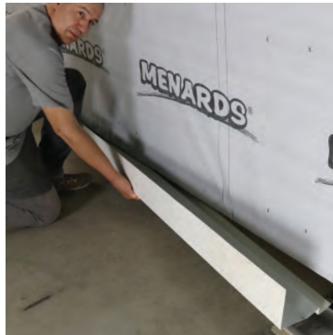
Bottom flashing installed over the WRB to cover foam.
