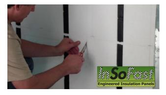
3. Then slice the foam like you are cutting a loaf of bread. It is okay to cut out a larger opening then the electrical box. You will need room to be able to work with the wiring.
