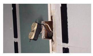
15. Once the drywall is installed over the InSoFast you may find that the electrical box is ½" to deep. This can be easily fixed.
