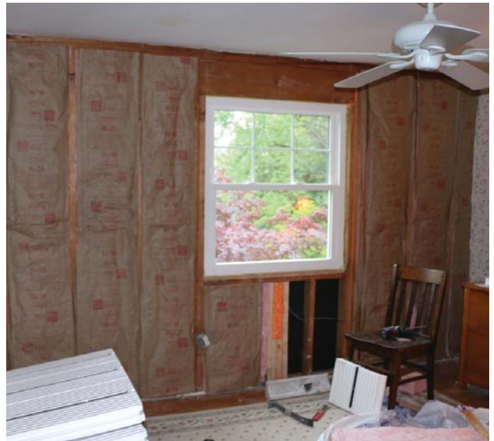
New fiberglass has been installed in the cavities.
