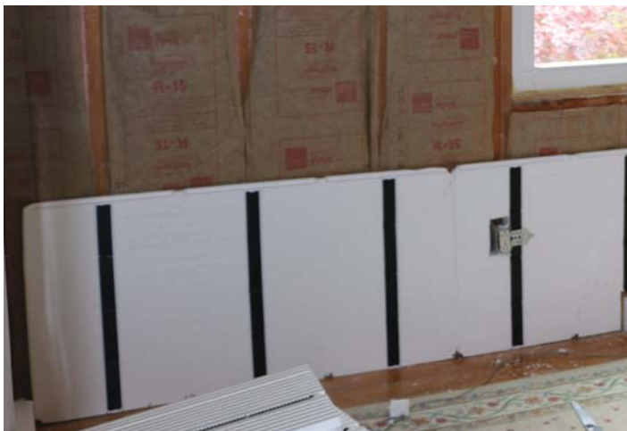
InSoFast panels line up with the wall studs.
