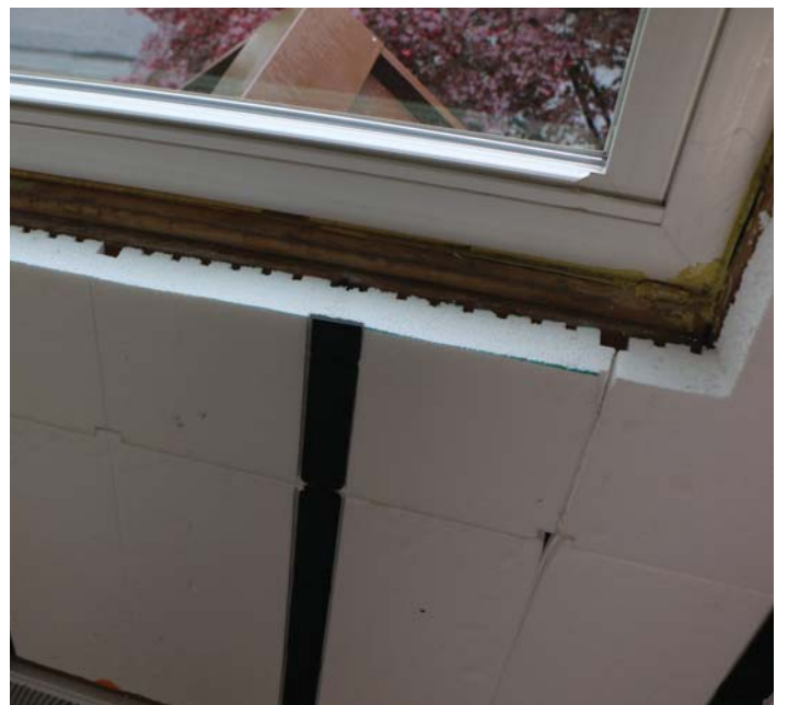
InSoFast panels installed over existing framing.
