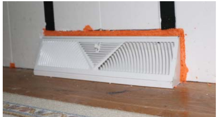
Heat register furred out flush with InSoFast panels
