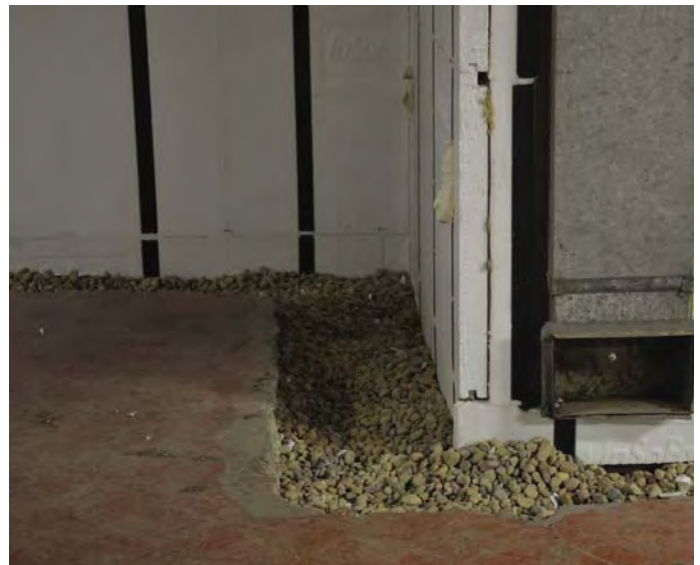
Drainage rock added for perimeter drainage.
