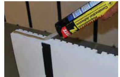
Glue bottom of top panel.
