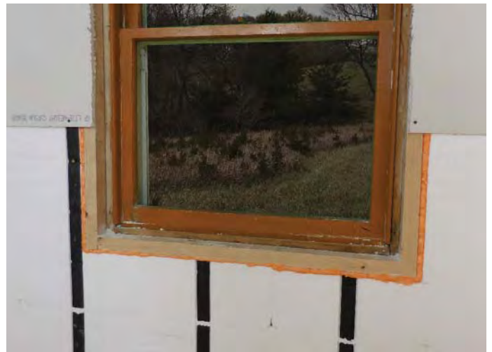
Seal around window to prevent air infiltration.
