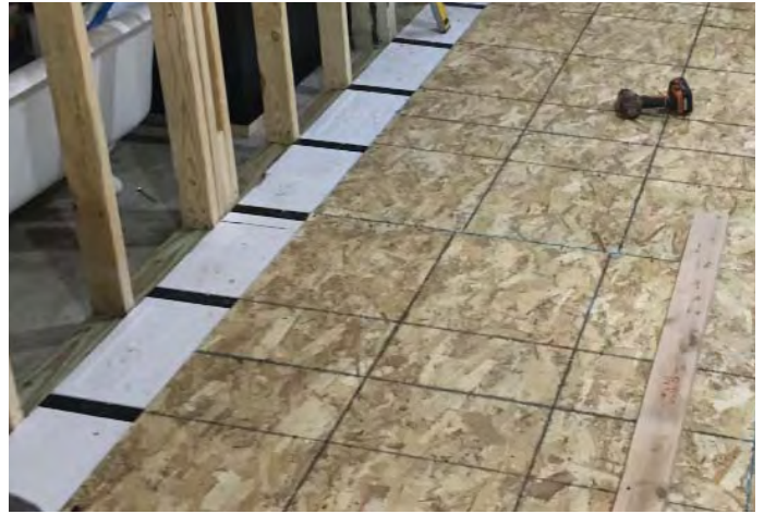
Butt up to load bearing walls.
