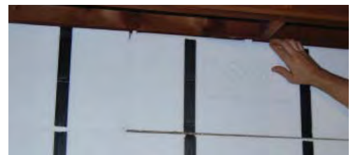
Set panel in place.
