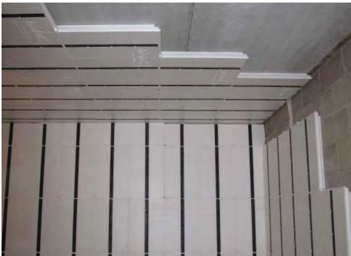
Panels installed in a staggered or running bond pattern.
