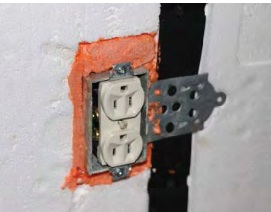
Face mounted box secured to stud.
