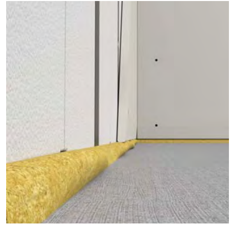
Seal the bottom of the wall.
