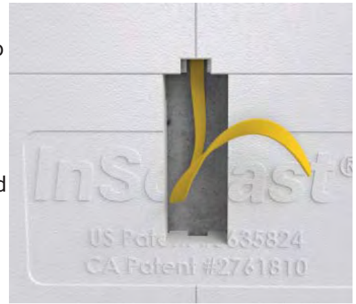
Cut out foam up to the horizontal raceway.
