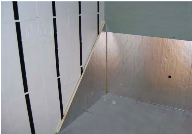
Add sheet foam over top InSoFast panels for increased R-Value.
