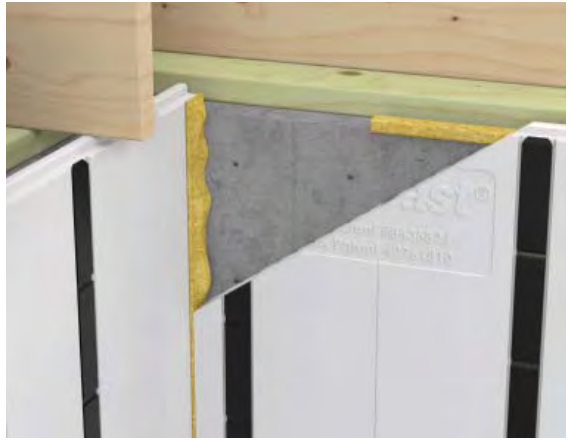
Use spray foam in the corner and at top of the wall.
