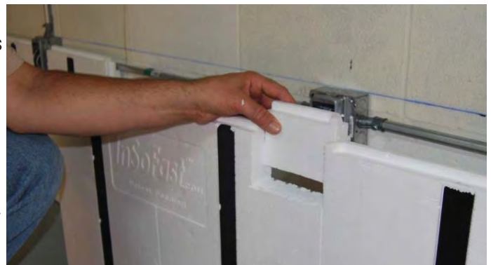
Cut out foam for existing conduit.
