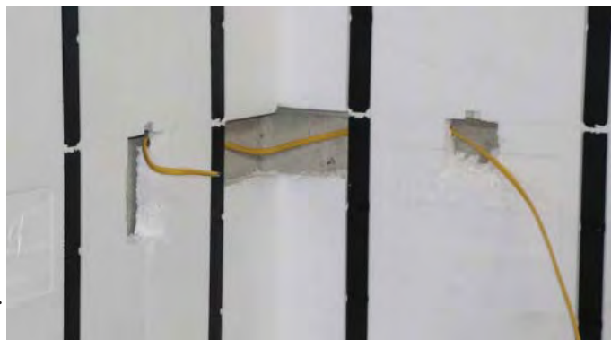
Cut out foam to run wiring around the corner.
