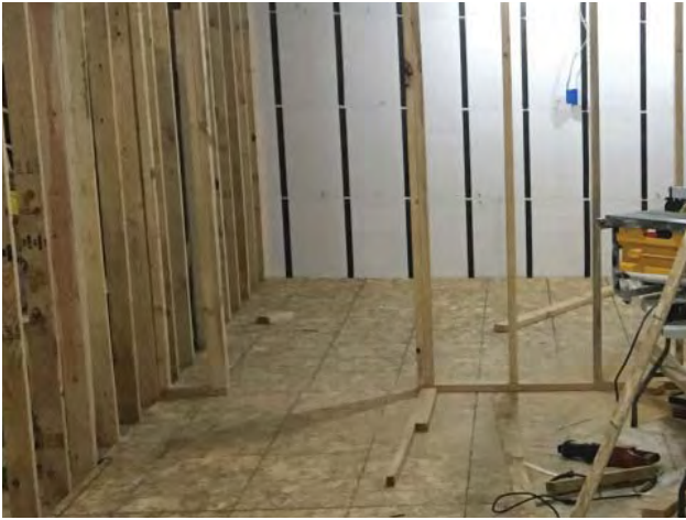
Non-bearing interior partition wall.
