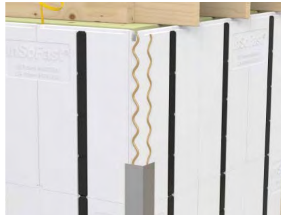
Use adhesive to adhere the metal corner flashing.
