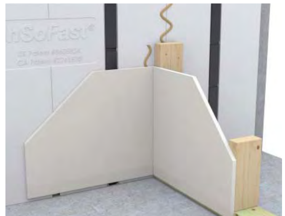
Use adhesive in the corners of intersecting walls.
