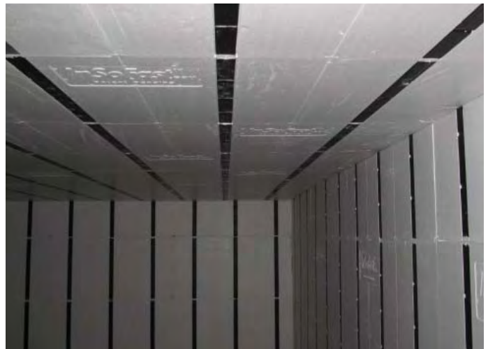
Ready for drywall. Allow adhesive to fully cure.
