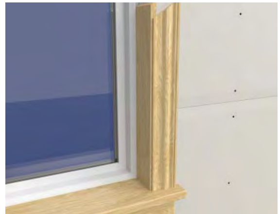
Install extension jambs and window casing.
