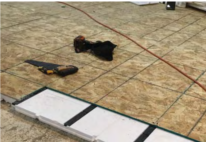
Line up end seam over InSoFast stud.
