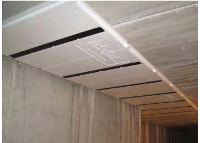
Install ceiling panels first.
