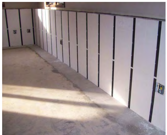
New concrete poured up against panels.
