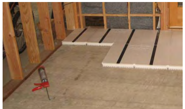
Glue down installation.
