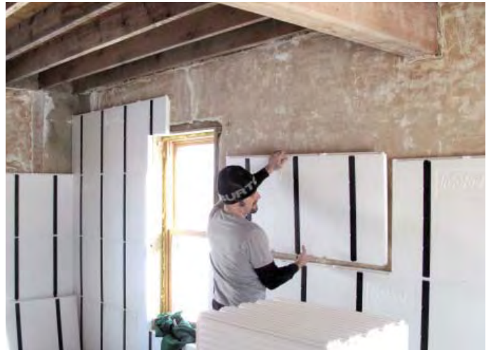
Alignment notches keep studs aligned.
