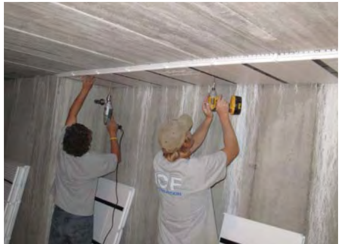
Panels installed with concrete screws.
