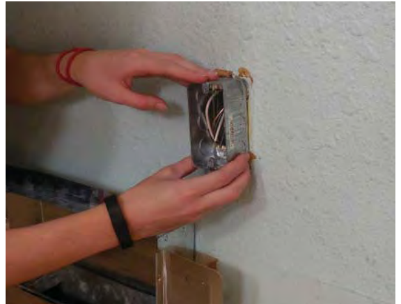
Use box extenders to accommodate new wall depth.
