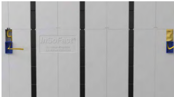
Horizontal raceways are 24" o.c.
