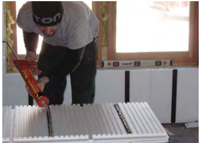
Apply a 3/8" bead of adhesive.
