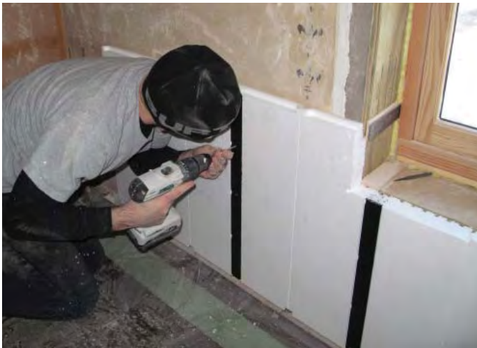
Optional mechanical attachment in the center of the panel.
