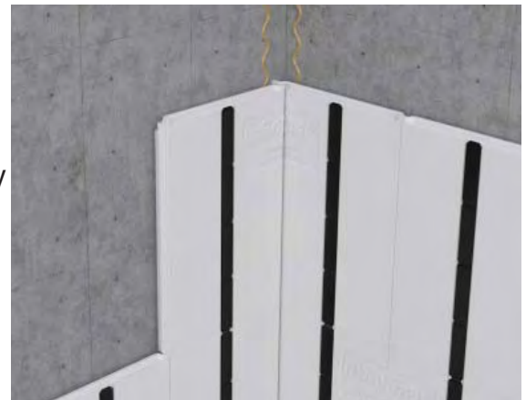
Cut 16" off the panel to start running bond.
