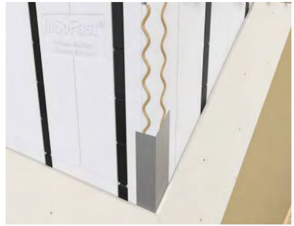
Screw drywall to metal flashing.
