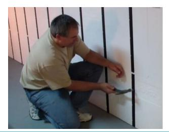
6. Use a hammer to drive the nail into the wall. Don't overdrive the nail. Tap the Perma-grip® fastener until securely seated.
