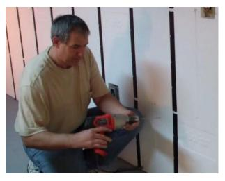
4. Here we will demonstrate installing a Perma-grip® nail. Use a Standard Hammer drill or Rotary Hammer drill to pilot a hole into the concrete wall.
