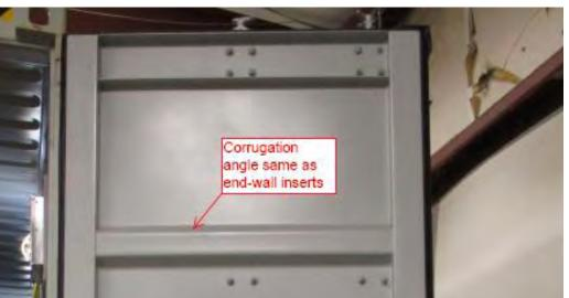
Center the EX 2.5 panel in a vertical orientation. It is important that the hard plastic studs do not center on the bumped out fasteners.
