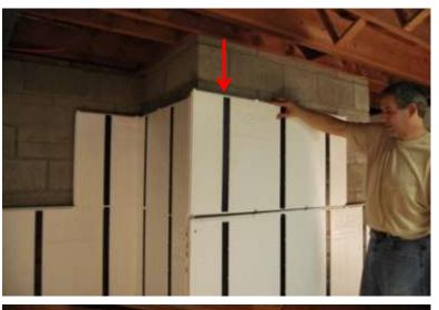
1. Once you place the last full row of panels measure down from the top of the wall to the top of the upper most panel. Measure, mark and cut the panel to fit.
