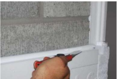
4. Remove the tongue with a sharp razor knife or saw.
