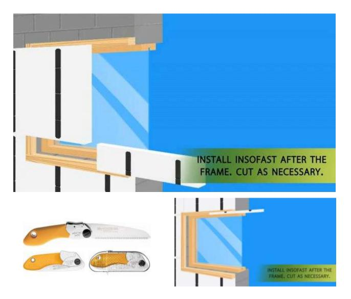
Now that the framing is installed cut the InSoFast to fit the opening. \*It is okay if you cut the panel  $\frac{1}{2}$ " shy of being tight, we will come back later and air seal around the opening with spray foam.
