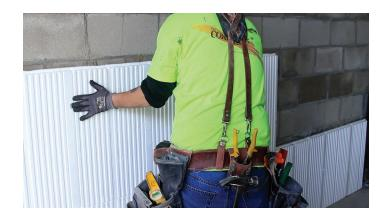
Fully insulated, embedded studs enable built-in attachment to walls and finishing materials. They are made from non-conductive composite material. The studs are recessed by a ½" of insulation to eliminate thermal transfer.
