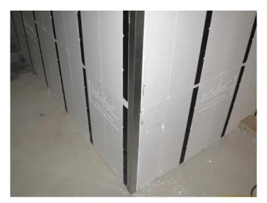
Apply beads of adhesive to the metal "L" angle, press into the corner then duct tape the corner until the glue sets.
