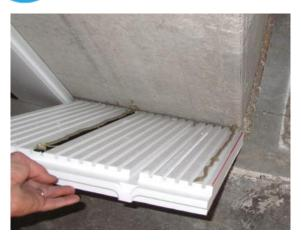
Apply a bead of adhesive directly on to the foam panel at the outside corner's edge and on all studs.
