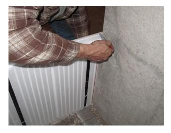
Mark and cut the panels about ¼" less than actual measurement needed so panels are not tight to the inside or outside corners, leaving a ¼" gap reduces the push out stress on the panels.
