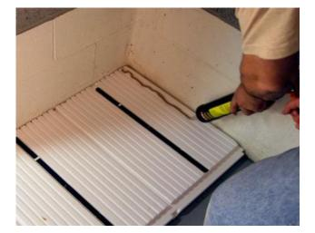
Apply a bead of adhesive directly on the foam on the backside of the InSoFast panel within 2" of corner cut.
