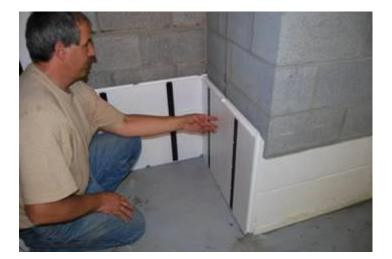
Leaving a ¼" gap reduces the push out stress on the panels so they remain flat and tight to the wall.
