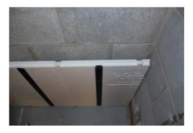
When you cut an InSoFast panel to fit into a corner the cut panel continues-turns or wraps around the corner.
